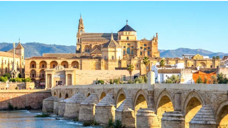
Historic Centre of Córdoba
